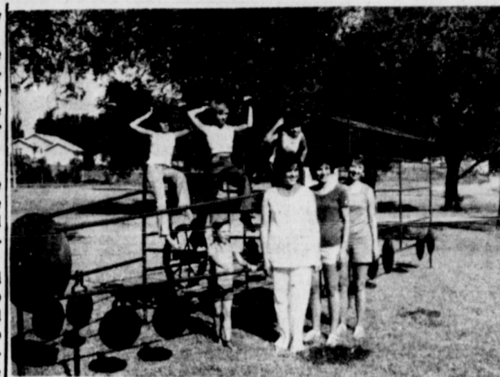
This is the Beta Sigma Phi Express built by George Martin's Ag Class and placed on the playground at the City Park Monday afternoon. Money from the Queen of Hearts Ball was used for material and it is the hope of the group to continue park improvement from other activities. Shown here are: Top, L to R—Gina Spier, Tracy Waters, Brigett Spier; Lower — Deanya Waters, Susan Henson, Pres. Darlene Spier, Past. Pres., Thelma Waters, Park Improvement Chairman. Staff Photo
