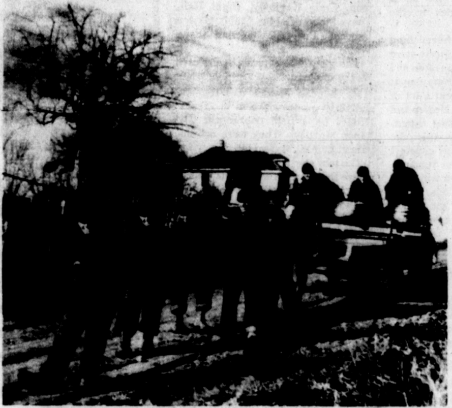
Early crews, like this one stringing lines in Kansas, built lines on an "assembly line" basis. A succession of workers went along country roads surveying, dropping poles and hardware, digging holes and setting poles, then stringing lines. This REA innovation was one of those which helped cut the cost of building rural lines to a third of what they had been only two years earlier.
