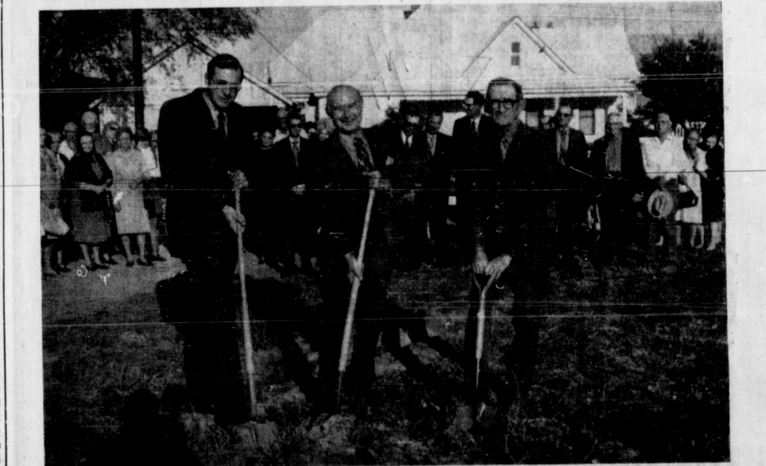
Ground breaking Ceremonies for a new Church of Christ building were held Tuesday morning on the lot where the new construction is to be located north of the present church. Shown turning the first spades of dirt, left to right, Tom Waters, local minister, Arling Cordell, chairman of the building committee and Robert C. Jones, former local minister and chairman of the finance committee. Members of the local church are looking on. —Photo by Saye's
