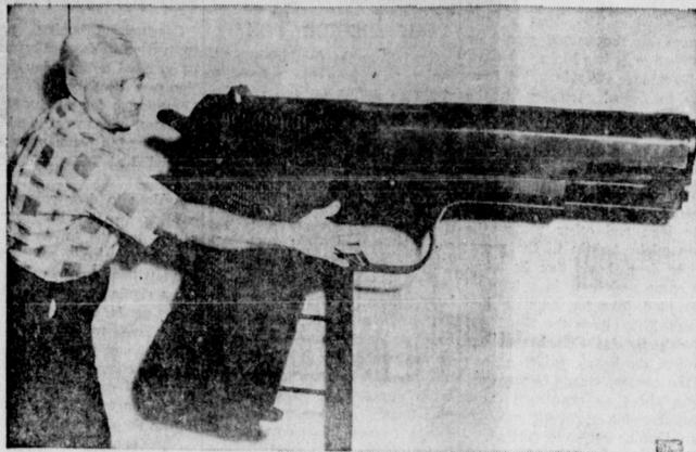
BIG BOOMER—Designer Raymond Hammond sights in on a plastic model of a .45 caliber automatic pistol at the Training Aids Center, Ft. McClellan, Ala. The model is 42 inches long, 10 inches high and weighs more than 40 pounds. It can be field stripped and reassembled in the same manner as the actual weapon. The giant replica is used as a training aid for instructors on the care and maintenance of the real weapon. (U.S. Army Photo by Pfc Rose A. Grzebyk)
