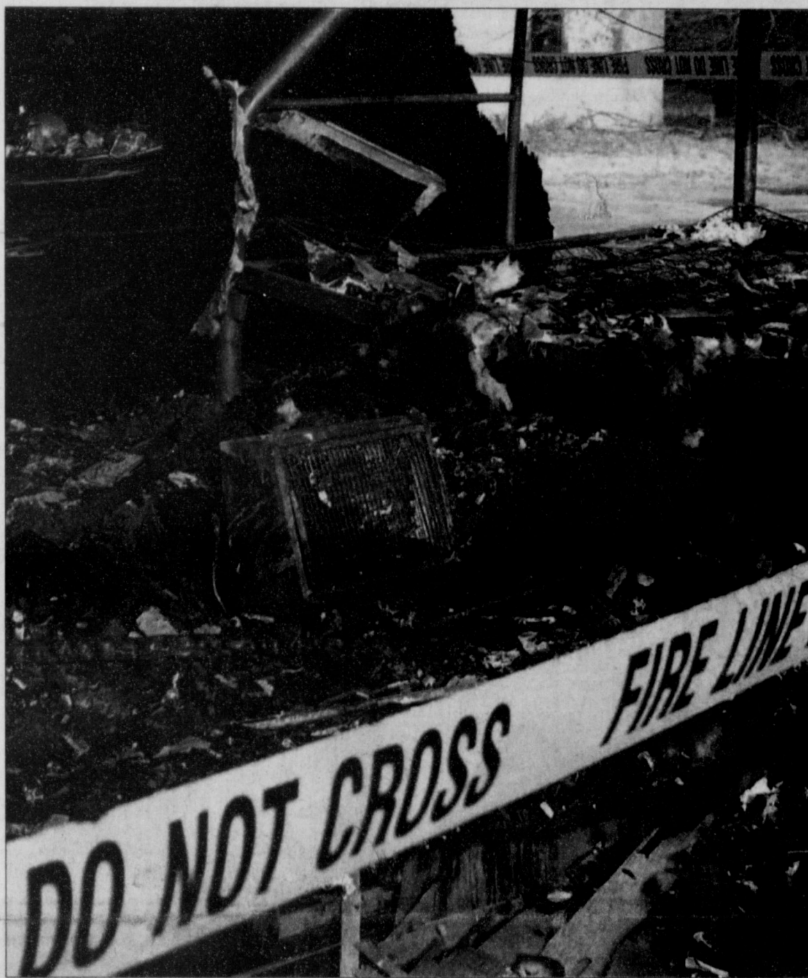
The charred remains of child's bunkbed stand just beyond a space heater that is said to be the cause of the fire that destroyed a local home last week.
