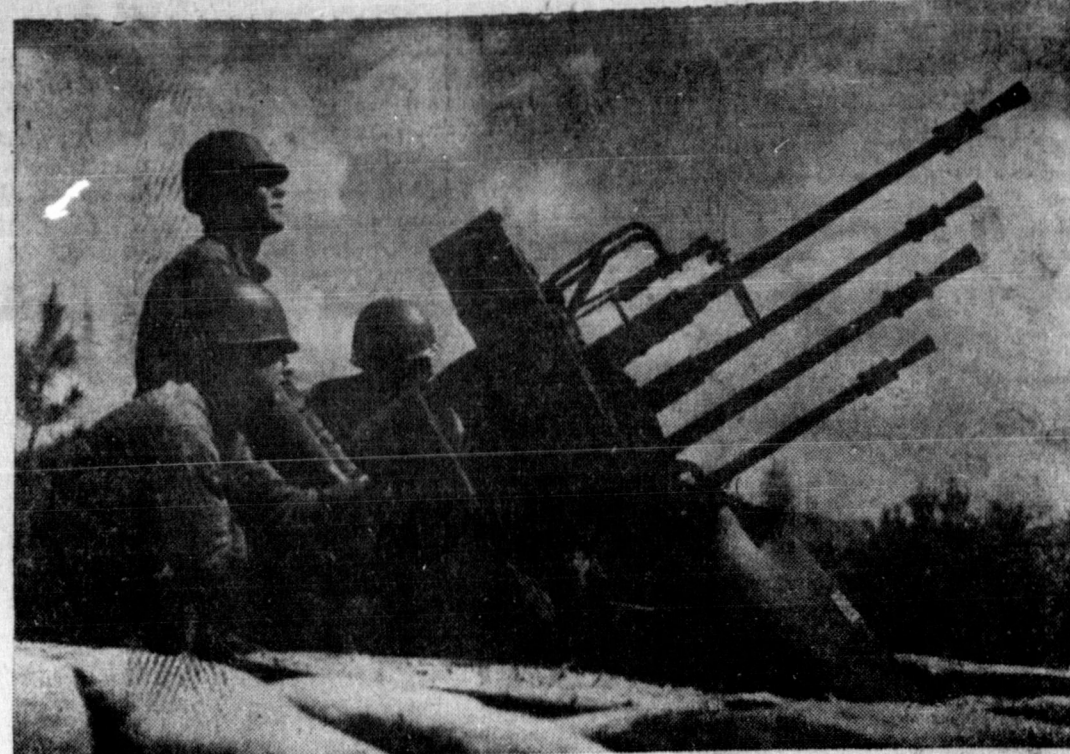
LEAD SPRAYER —When planes flew lower and slower during World War II, this anti-aircraft weapons system of four 50-caliber machine guns, towed or mounted on a tracked vehicle, proved to be a highly effective mobile defender of front line positions. With the advent of the jet age and combat in Korea, soldiers merely depressed the four barrels and found themselves with a tremendously lethal anti-personnel weapon, capable of firing 2400 rounds a minute, for cutting a swath through mass waves of attacking Communist troops.
