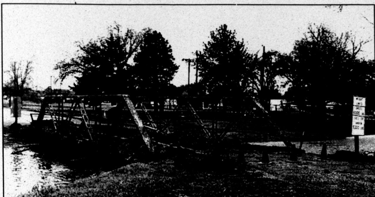
High waters washed over the bridge on Seventh Street at the City Park last week, covering it with grass and debris.
