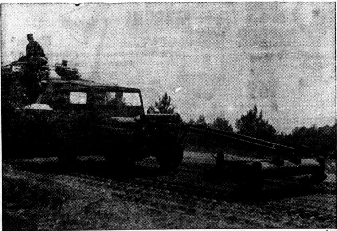
MINE DETECTOR automatically stops the jeep it proceeds when it locates a land mine. The hydraulically controlled detector covers a 6-foot swath directly in front of the vehicle and can be moved to both sides to cover the road shoulders. This jeep mounted mine detector is a product of Willys Motors, Inc.
