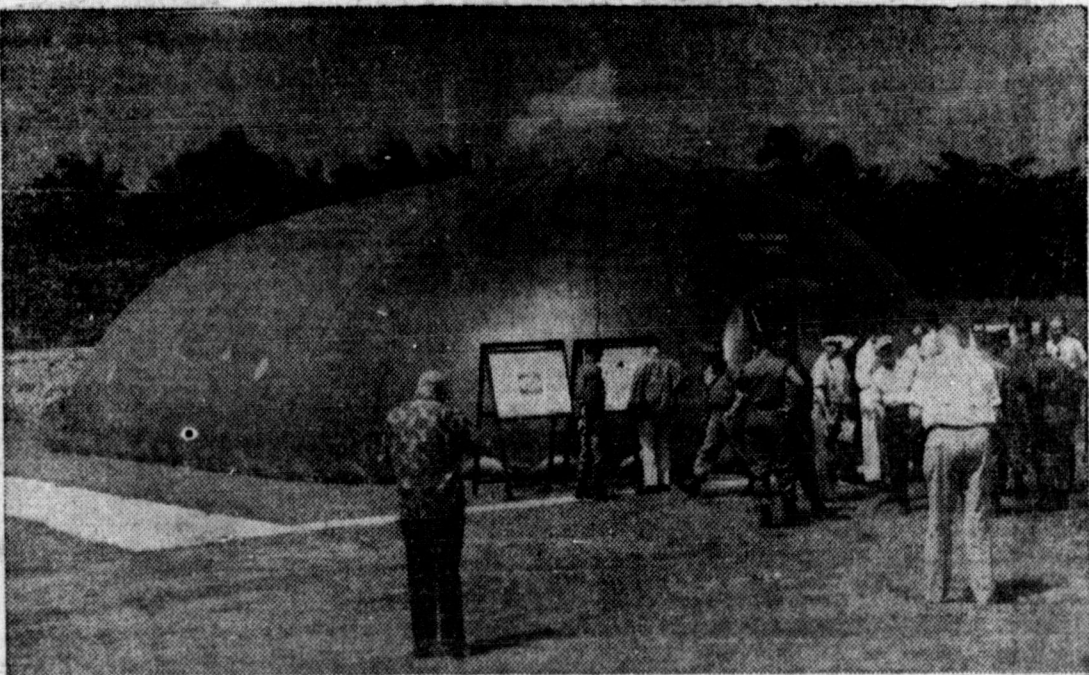
ENORMOUS AIR-INFLATED, AIR-TRANSPORTABLE SHELTER used by STRAC for briefings at Exercise BIG SLAM/PUERTO PINE held in March. Developed by Army Quartermaster Corps, the shelter when fully inflated is 40-feet wide, 80-feet long and 15-feet high. When deflated it makes a package four by five feet and weighs less than 700-pounds. Made of vinyl coated nylon, it attains and maintains its shape through high volume, low pressure air supplied by power blowers. The shelter has no center supports, poles or other obstructions to hamper movement within.
