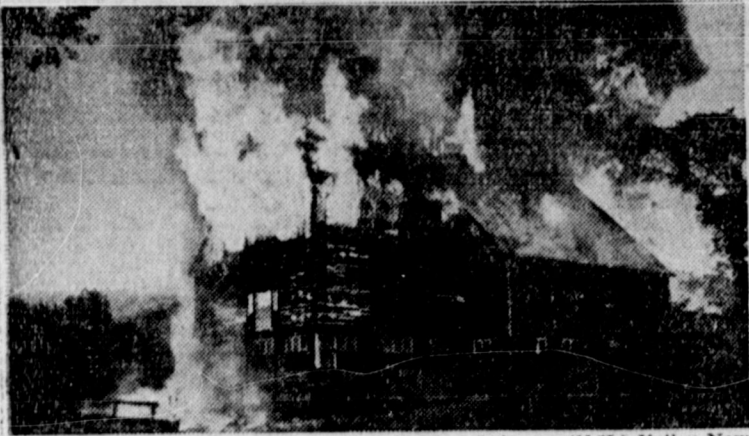
This $50,000 barn with contents value at $10,000 burned in West Hartford, Vt., when a pitchfork broke an electric light bulb and set fire to hay in the loft. It was a complete loss—not even insured. The nearest water supply was a brook 800 feet distant; yet there was no hose, no pump, and no fire extinguisher, and the farmer wasted 20 minutes trying to put out the fire before calling the firemen.
