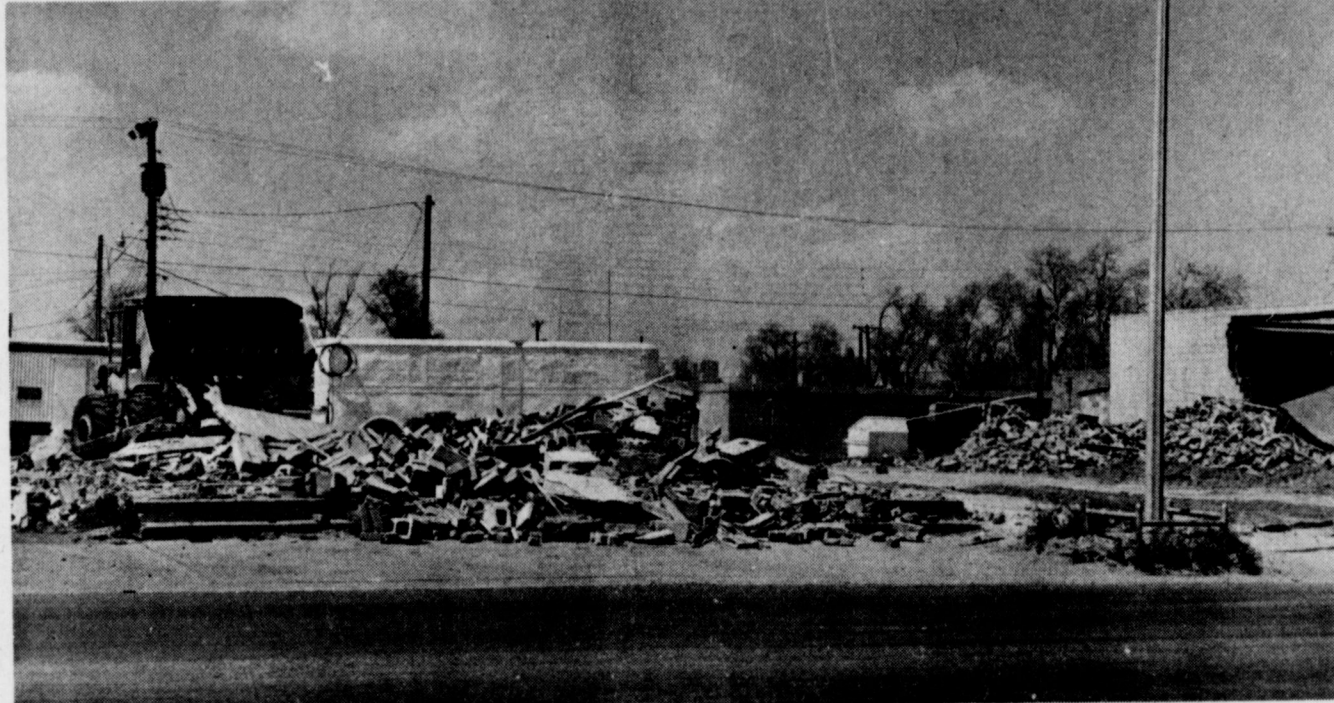
BUILDING DEMOLITION UNDERWAY . . . Workmen began late last week demolishing several buildings in the 200 block of South First Street. The buildings formerly were occupied by a cotton buyer's office; the Alcoholics Anonymous meeting room; a small
