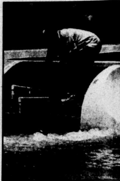
A.J. Moffit turns on the valves to the waterslides at Thunder Junction which connected the park to the city water main on Tuesday, August 25, 1998.
