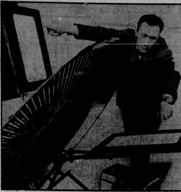
TRI-DIMENSIONAL WHEEL —Something new in the projection of third-dimensional movies has been invented by Alberto and Adriano Betti. Instead of giving spectators glasses, the Roman twins synchronize a projector with this revolving glass disc which has alternating mirrors and transparent segments. Two images are projected through the disc, one reaching the viewing screen, left, while the second is reflected by the mirrors to another screen, right, and from this back to the viewing screen, giving a third dimensional appearance to the movie.
