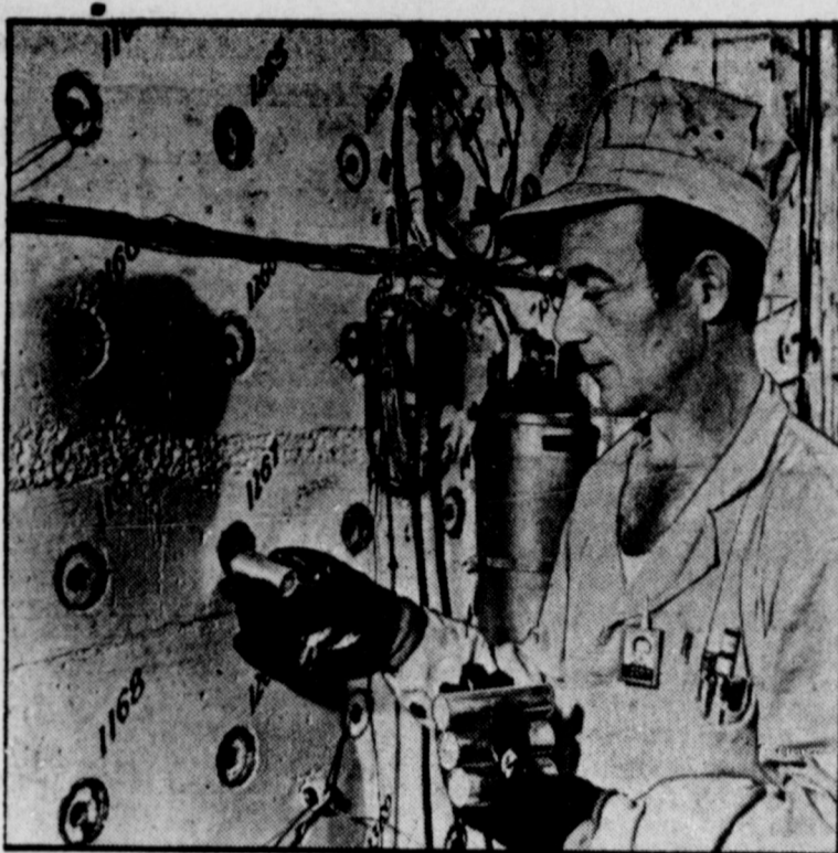
FEEDING TIME AT OAK RIDGE — A workman places an aluminum-jacketed uranium slug in a fuel channel opening of one of the graphite reactors that make up the atomic pile at Oak Ridge, Tenn. The natural uranium slugs, like the one being inserted above, weigh 2.57 pounds each and are four inches long.
