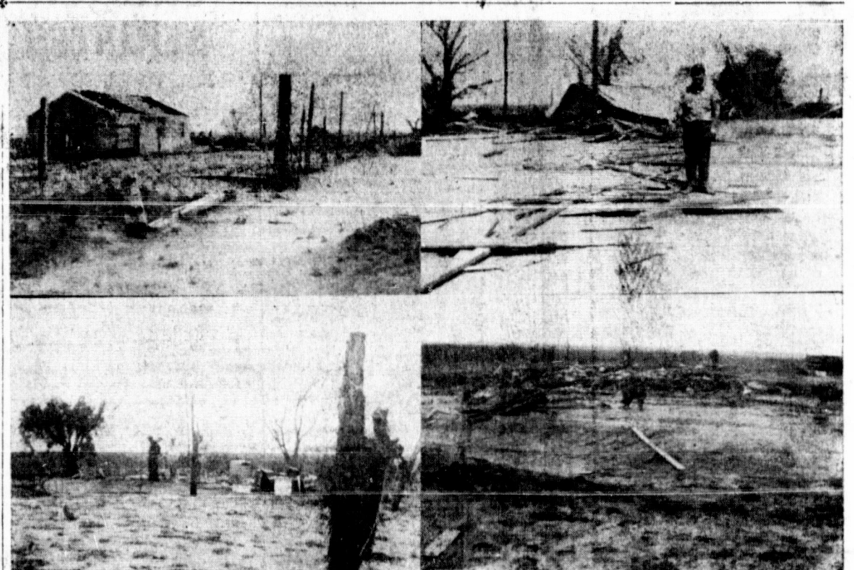
Pictured top left, O. L. McBrayer home on Porter ranch; Joe Shadle standing among the rubble of outbuildings on Tam Shadle place. Bottom—pictured at left is group of men standing where the J. D. Jones home stood before the storm; to the right is where the Jones house was washed. The dog in the picture went through the storm unhurt. After taking the first picture he walked out to the pile of rubble as if to show us this was all that was left.
