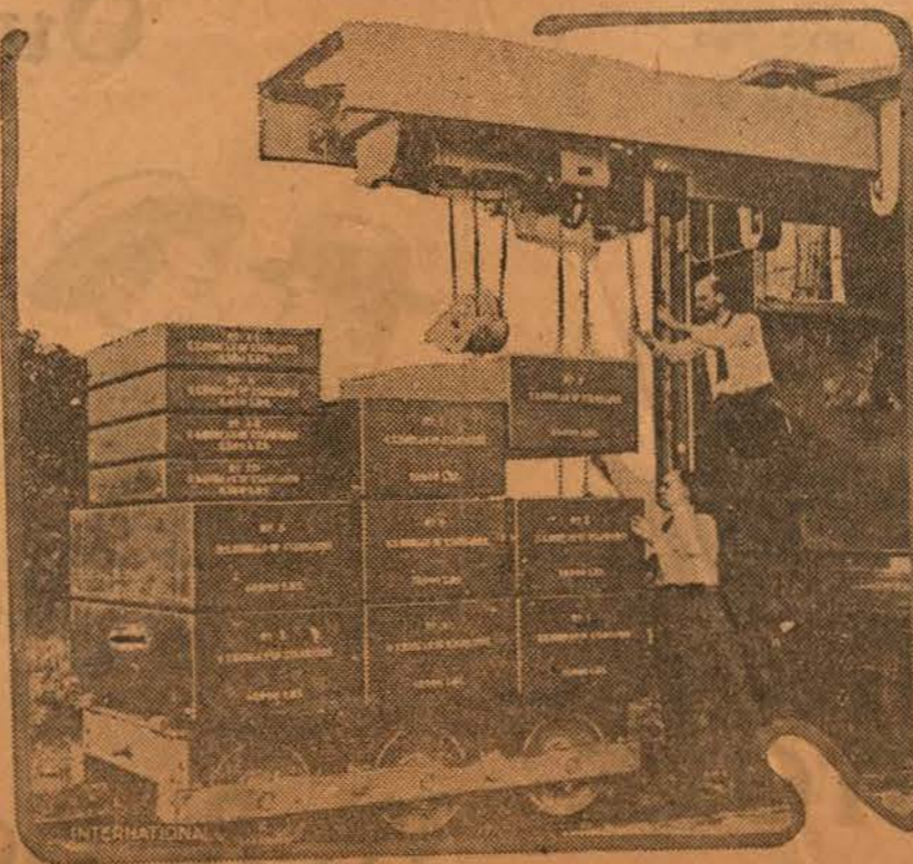
A railroad track scale testing car of the national bureau of standards, Washington. The car is fitted with weights of 10,000 pounds each, and is sent about the country to test railroad track scales. It also sets the standard by which is calibrated the test cars of the railroad companies.
