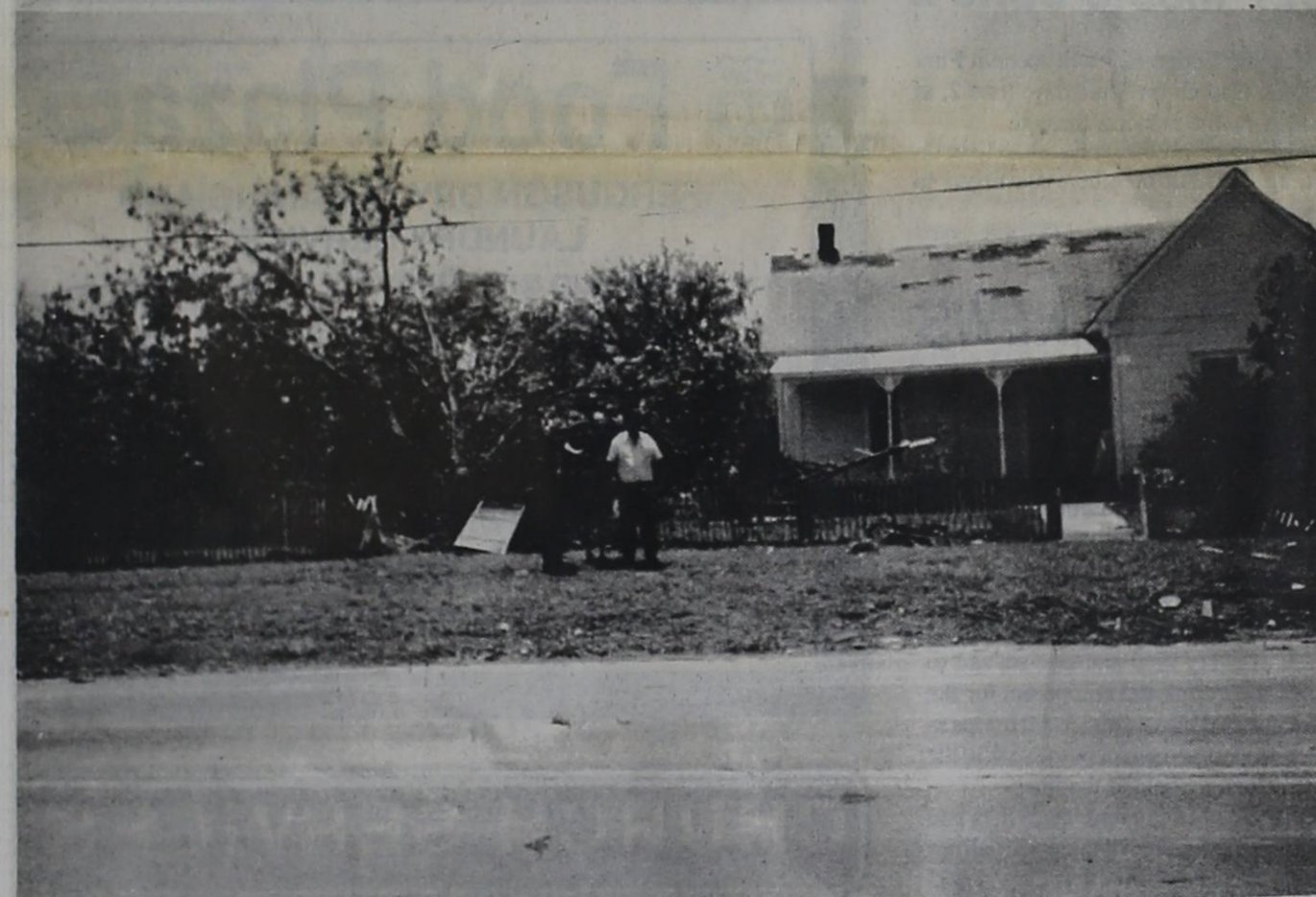
HOWARD HOUSE DAMAGED — Shingles were blown from the roof, the picket fence and special gate are down, and a large tree was uprooted in the yard of the historic property.
