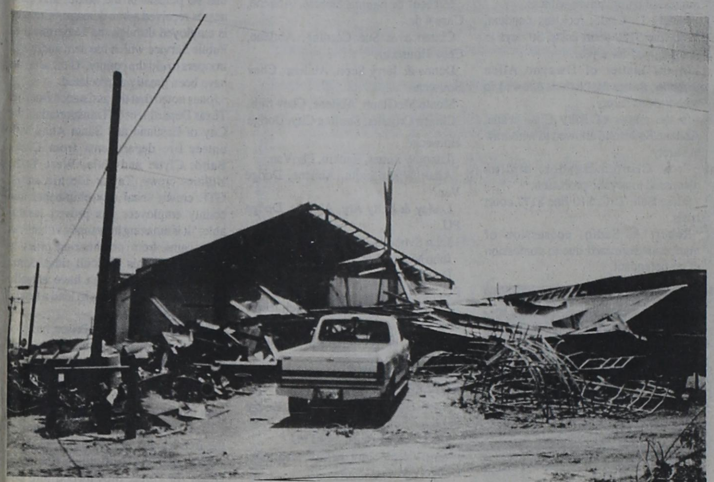
LAWRENCE FARM & RANCH SUPPLY, INC. WAREHOUSE DESTROYED
