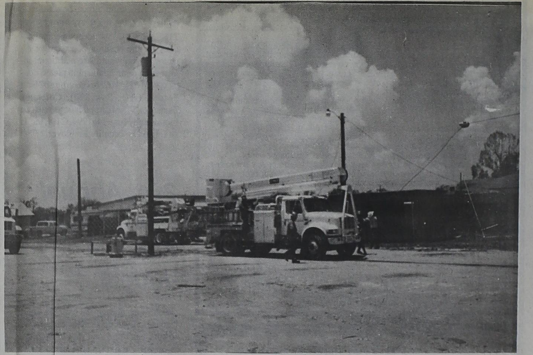
WEST TEXAS UTILITIES CREW WORKING NEAR ODOM'S MOTEL
