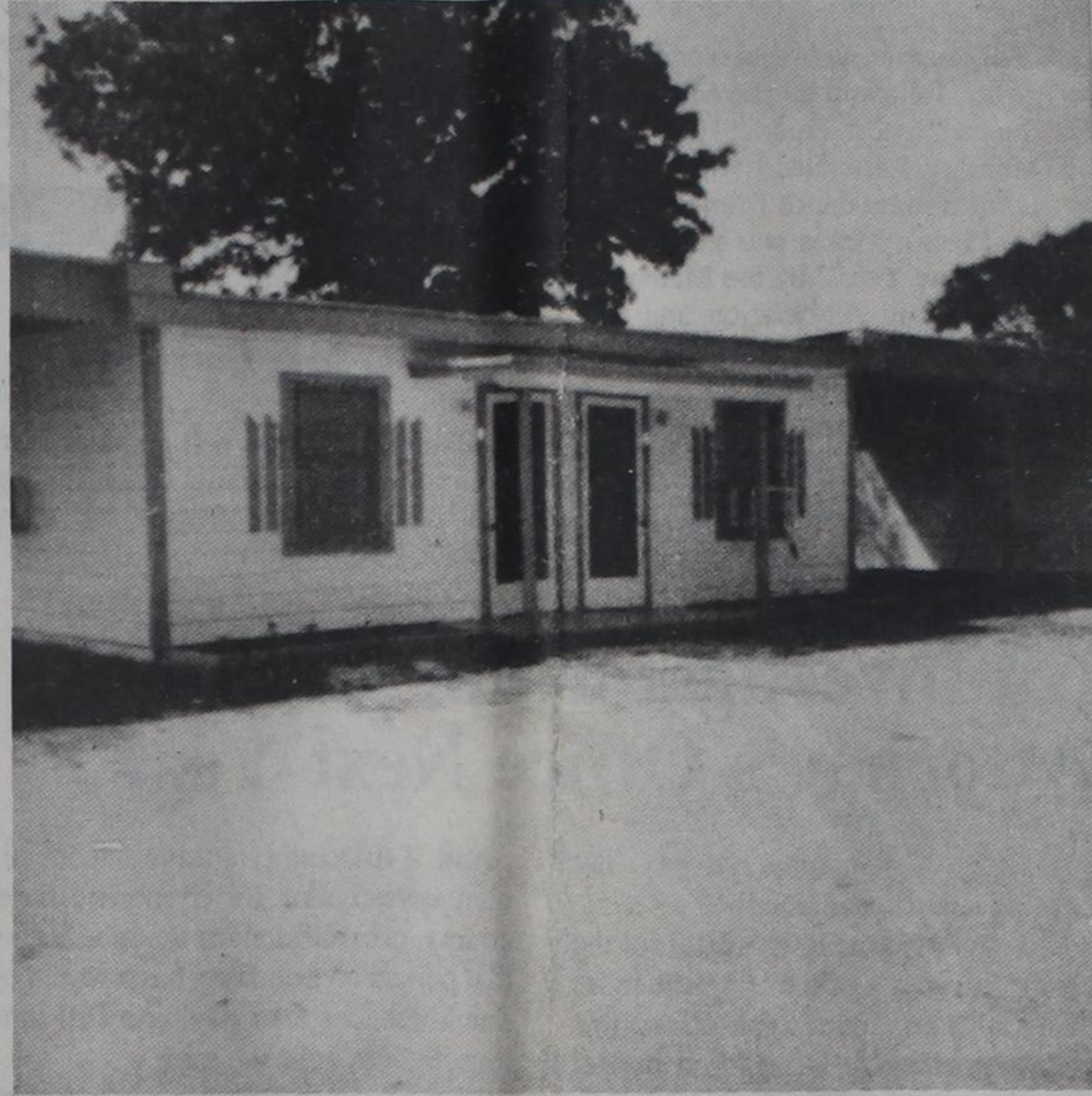
REMODELED — The rooms at Country Inn Motel reflect country
