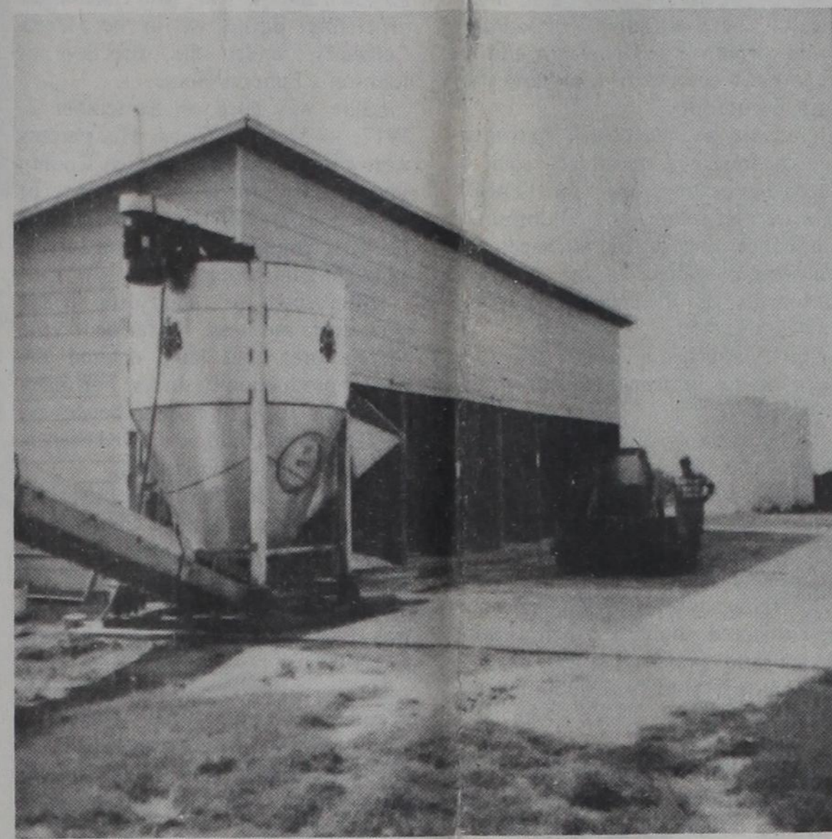
BLENDER AND BINS — A look at the eight storage bins and massive fertilizer blender.
