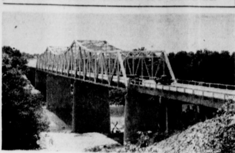
The Texas State Highway Department's newest truss span bridge is this $265,000 structure spanning the Brazos River on U. S. Highway 67, fifteen miles west of Cleburne, Texas, in the Glenrose hill area. The 1,200-foot bridge contains 750 tons of structural steel supplied by Virginia Bridge Company, U. S. Steel Corporation subsidiary. Completed May 31, 1947, after 208 working days, the bridge is an important span in one of the nation's principal transcontinental highways. Harry Newton, Graham, Texas, was the general contractor and steel erector was John F. Beasley, Dallas.
