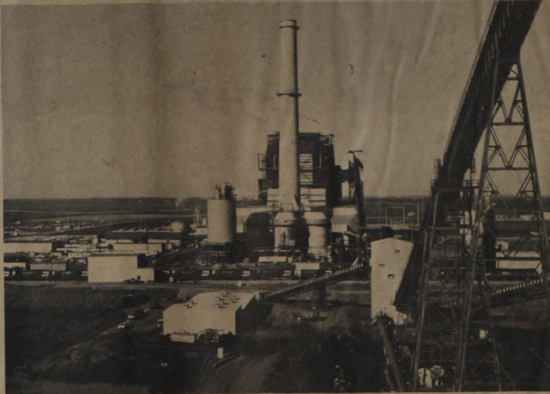
NEW WTU POWER PLANT — The Oklaunion Power Station near Vernon
