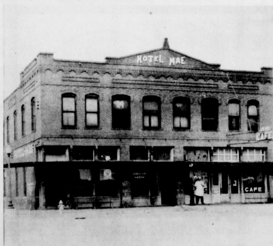
TO BE RENOVATED IN NEAR FUTURE — This old building is known as the Mae Hotel, located on the
