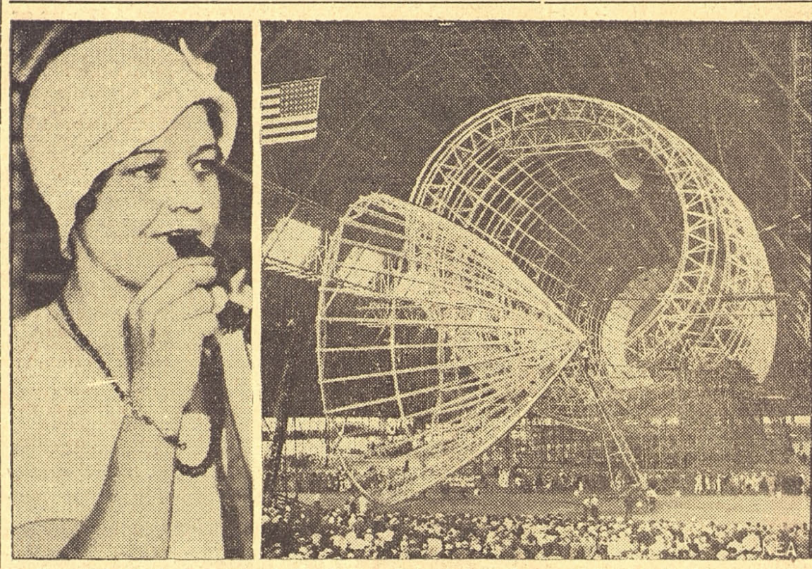
The U. S. navy's mammoth new airship, the U. S. S. Macon, entered the final stages of construction at the Goodyear-Zeppelin dock in Akron, O., when its 75-foot bow was lifted into place with elaborate ceremonies.
