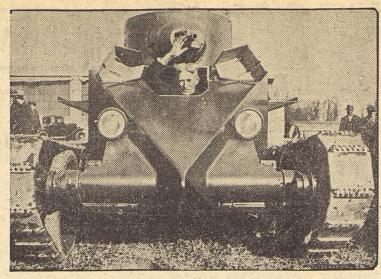
Walter Christie, automotive engineer, waving from the circular door of his new super-tank, which was demonstrated to military authorities at Linden, N. J. The tank can attain a speed of 75 miles an hour on an open road. With the caterpillar tracks it can speed across any rough country at 45 miles an hour. It possesses %-inch armor and carries a one-pound cannon and 30caliber machine guns with 2,100 rounds of ammunition.
