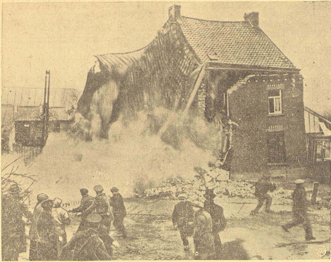
In the remarkable photograph above, the camera caught the full tragedy of a disaster that left 200 Belgians of the village of Courcelles homeless, when a subterranean landslide caused buildings to collapse without warning. Terrified passersby are shown fleeing from the sudden crashing avalanche of bricks and roof tiles.
