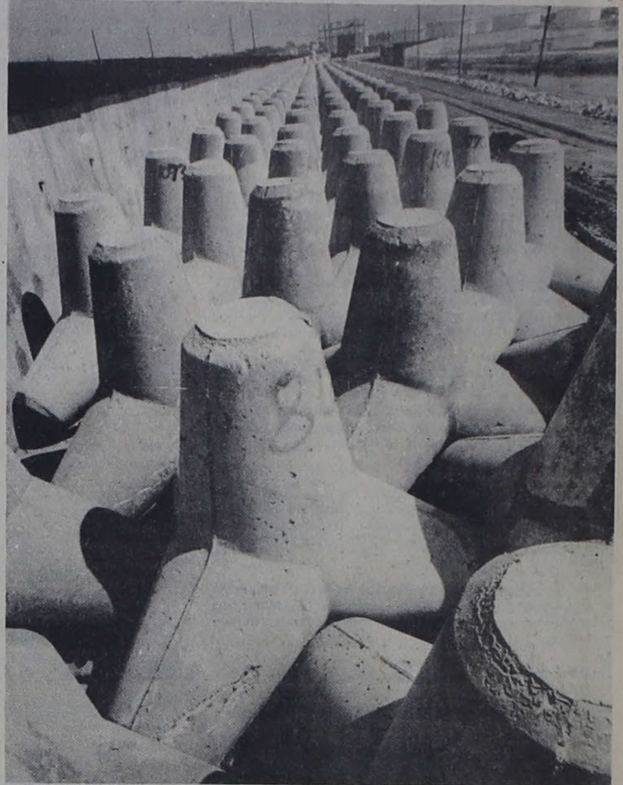
TETRAPODS —Shaped like children's playing jacks, these concrete "tetrapods" are part of a $12 million flood-protection project for the dock area of Exxon USA's Baytown, Texas, refinery. In the event of a hurricane, the tetrapods would break up the force of heavy waves which might sweep out a small bay nearby, cross the road pictured at right and then crash into the seawall at left. Two more layers of tetrapods are being placed on top of those pictures for a total of 1,650 tetrapods bordering a 1,200-foot section of seawall. Each of the four-footed (definition of "tetrapod") objects weighs two tons and stands about five feet high.
