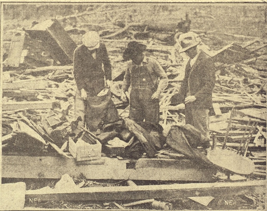
Bales of hay scattered amid the wreckage of a partly demolished home in Northport, Ala.
