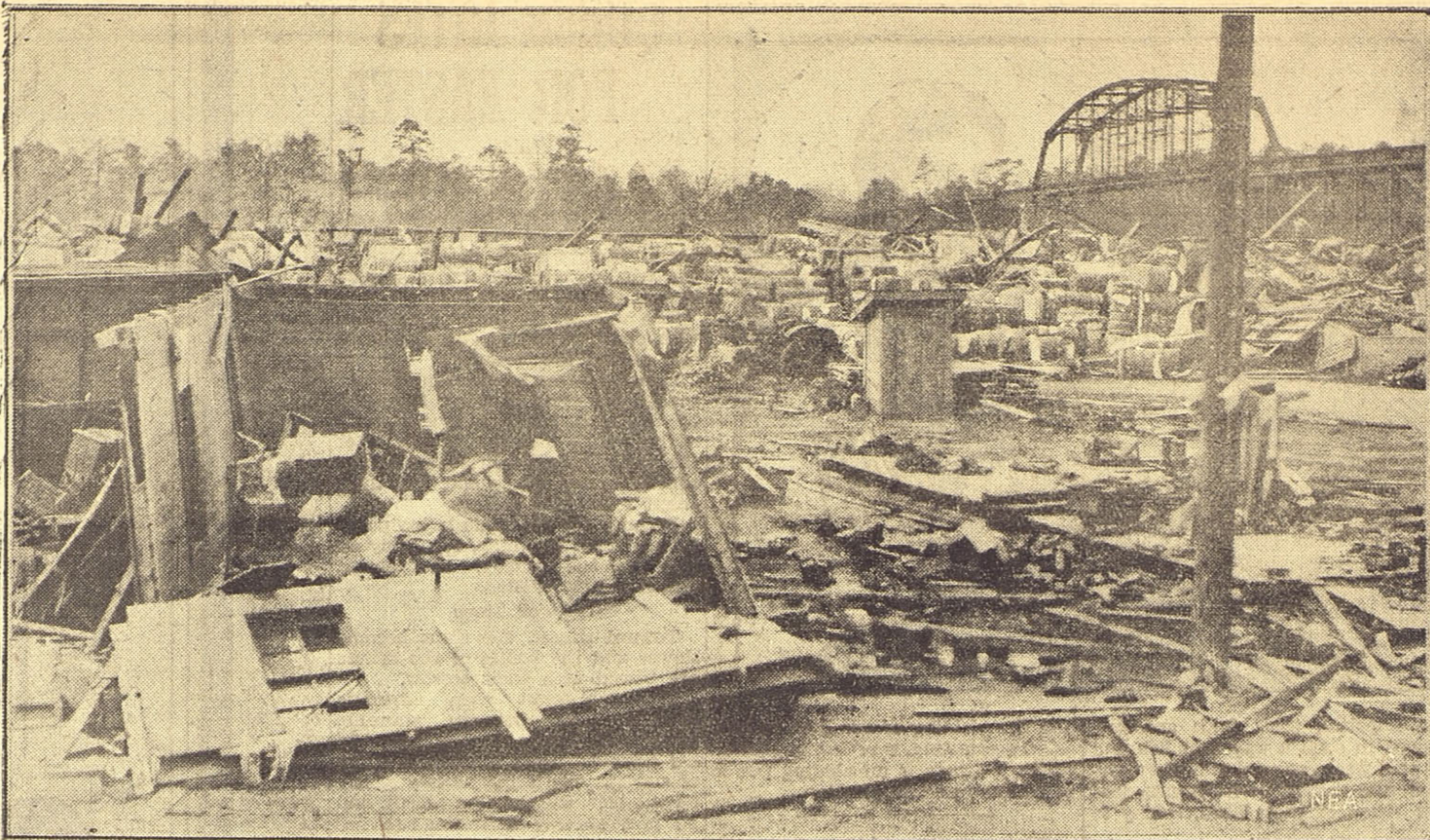
Scene of wreckage wrought by storm in Northport, Ala.
