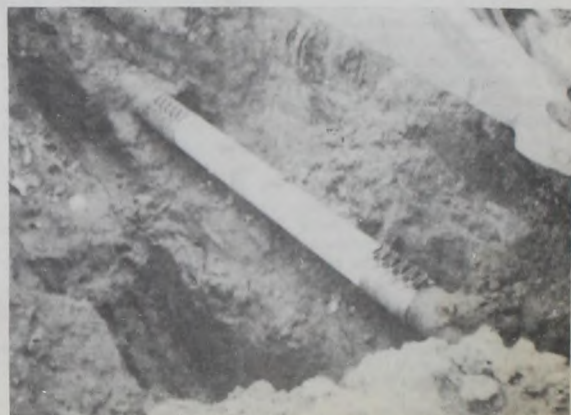
WATER MAIN LINE REPLACED AT RANCH ROAD 1065 AND JONES STREET SATURDAY.
