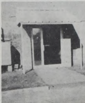
CHURCH GETS PORCH A new cover over the east door of Turkey Methodist Church was installed to keep rain from blowing in under the door. Constructed and installed by Don Turner.
