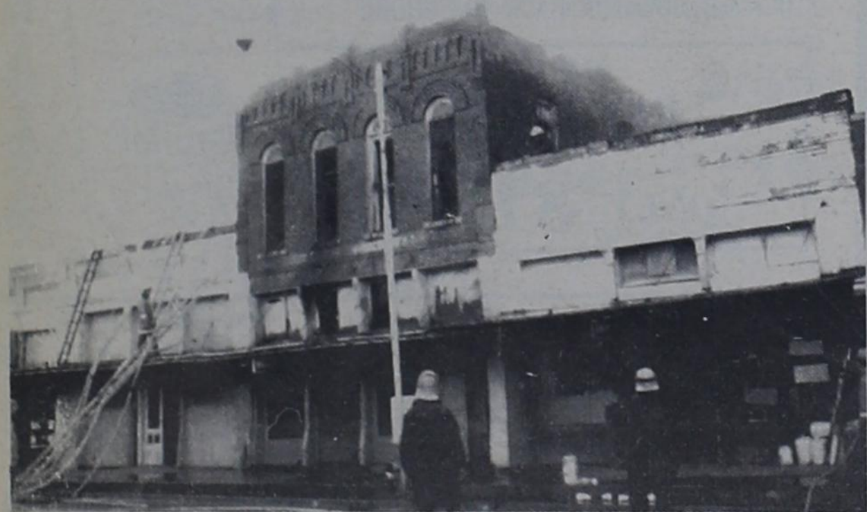
BAIRD-CLYDE FIREMEN —Keeping watch after fighting 5 hour blaze that destroyed Work's Dry Good store, Thursday, August 2, 1979. The fire began around 2:30 a.m.
