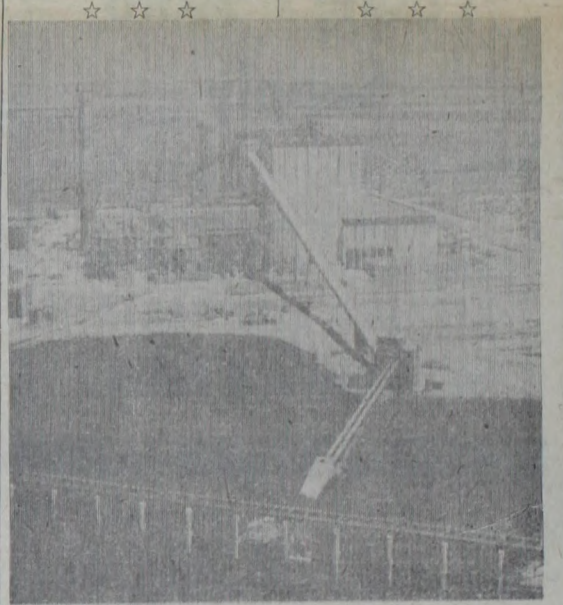
Low-sulphur western coal is the fuel for Southwestern Public Service Company's Harrington Station. Located northeast of Amarillo, Harrington Station is the new-
