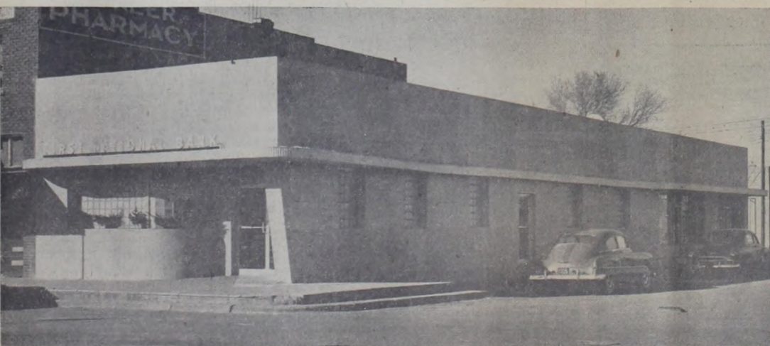
The above photo is the exterior view of our bank after the 1950 repairs.
