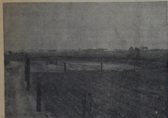
This waterway is a tributary of Kent Creek. Once a yawning gully deeper than the one pictured above, it will be seeded to wheat or rye as soon as possible. When the native grasses are established some grazing will be possible, and the owner, J. B. Baird, will be able to move machinery from one field to another without detouring the deep chasm. — Photo Courtesy Briscoe County News
