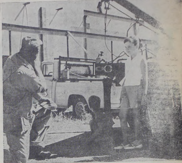
NEW FAIR BUILDING . . . Three young residents of the Panhandle South Plains Fairgrounds at Lubbock take special interest in a new building under construction. It will house what fair officials describe as the largest Children's Barnyard exhibit ever to be shown at the fair, which opens Sept. 23 for a six day run. Construction Superintendent J. I. Jenkins, at left is shown explaining the front of the building to Steven Lee (kneeling) and his brother and sister Robbie Lynn and Vickie Diane. The children's father, Albert Roller, is employed by the Fair Association.
