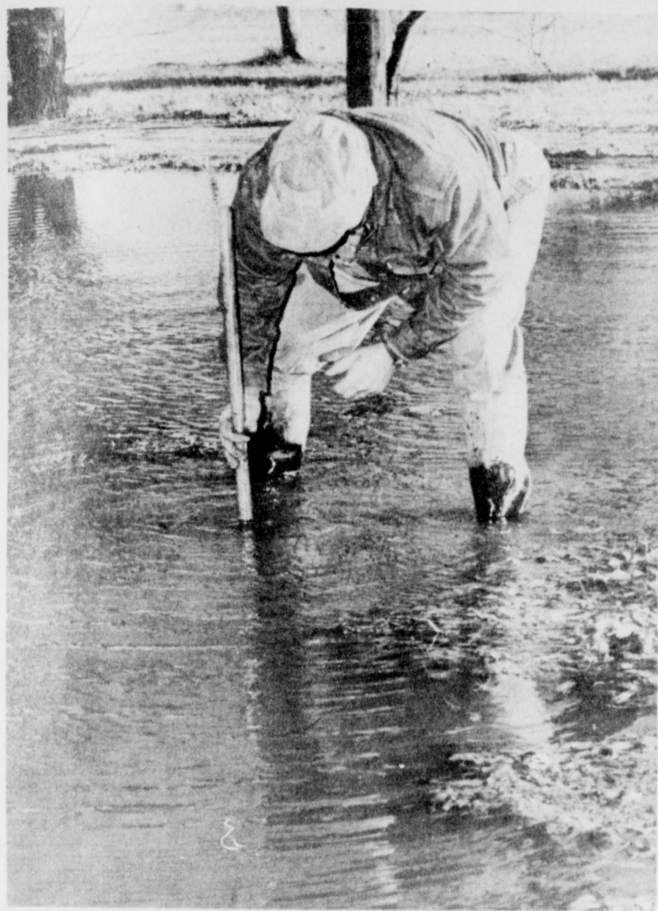
YARD INUNDATED -- A city worker probes underwater with a shovel to free debris from a drain pipe at a home near the intersection of North Jackson and West Washington. Ditches and yards were inundated when fire hydrants were opened to relieve pressure on aging water lines out of fix.
