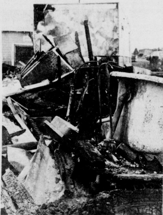
HOME DESTROYED - A charred bathtub stands juxtaposed amid the ruins of a Holliday home that burned Tuesday morning. Located on Southwest Avenue, the home was owned by Louise Conway Loyd. No one was injured in the blaze reported shortly after 8 a.m. Tuesday.
