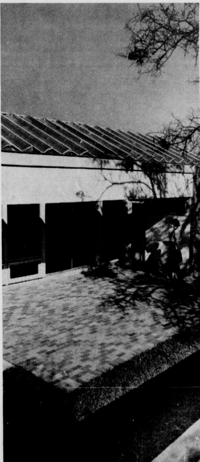
Texas Electric helps sponsor the Discovery '76 House at the University of Texas in Arlington. The sun's heat is used to run special heating/cooling equipment.
