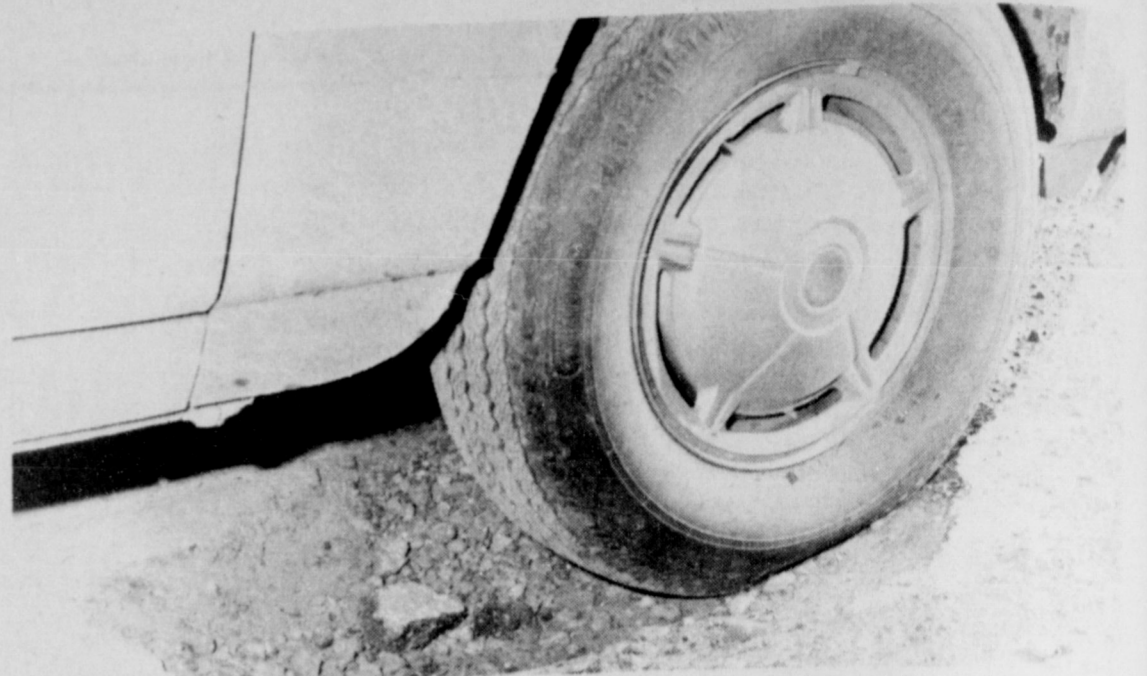
BUMPY RIDE —Street chug holes knocked out by last week's snow storm will inconvenience Iowa Park motorists for several weeks, city officials say.
