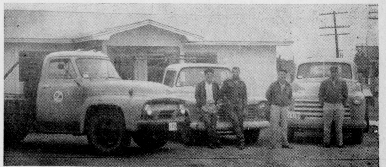
This picture points up three phases of Gary-Nees Lumber Company's operations in Iowa Park. First, the personnel which makes us a service organization. They are (left to right): L. A. Powell, Perry Johnston, Eugene Johnston, Homer Singleton. Second, some of the rolling stock which gets your materials to the job promptly and in good condition. And third, our new office building which makes doing business with Gary-Nees a pleasant experience.
