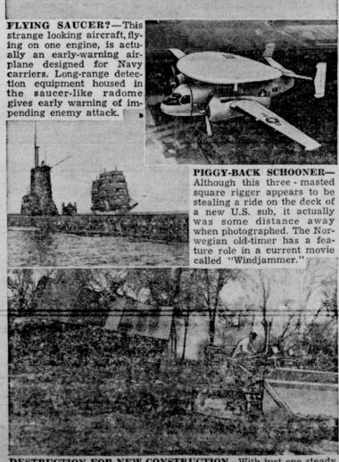
DESTRUCTION FOR NEW CONSTRUCTION—With just one stead; pull on the cable, this International Drott TD-9 Skid-Shovel topples a shack that stood in the way of progress for the new Atlanta, Ga., expressway. After the tractor had pulled over the shack, it returned and loaded out the debris.
