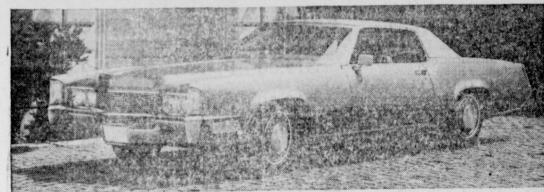
The 1969 Cadillac is dramatically restyled to look lower, wider and longer. The Fleetwood Brougham (top) shows the new dual horizontal head lamps and the combined parking and cornering lights wrapped around the leading edge of the front fender. The familiar cross-hatch grille features horizontal and vertical bars in a "floating fin" effect.
