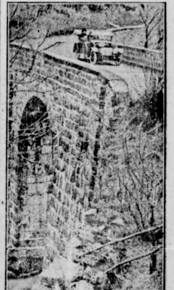
Substantial Stone Culvert.
