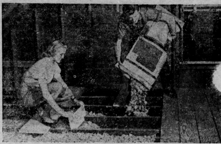
Man-and-wife team pour mineral wool insulation into attic floor.
