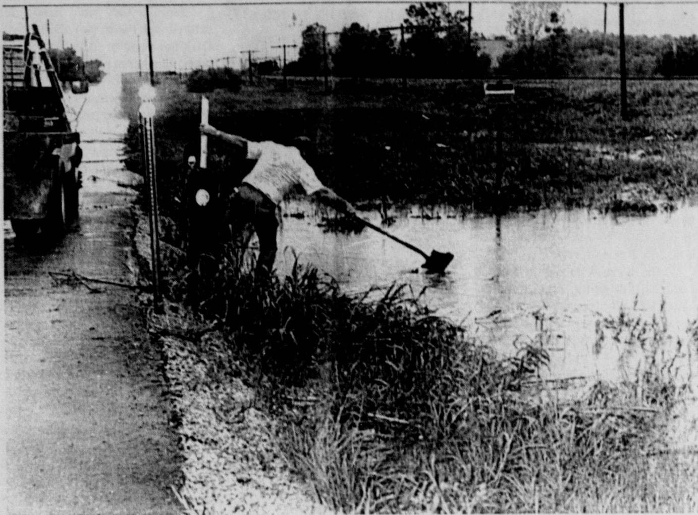
DONALD POTTER CLEARS DEBRIS FROM CULVERT ON SMITH ROAD ... after heavy rains floated railroad ties, felled trees and trash under and over the roadway.
