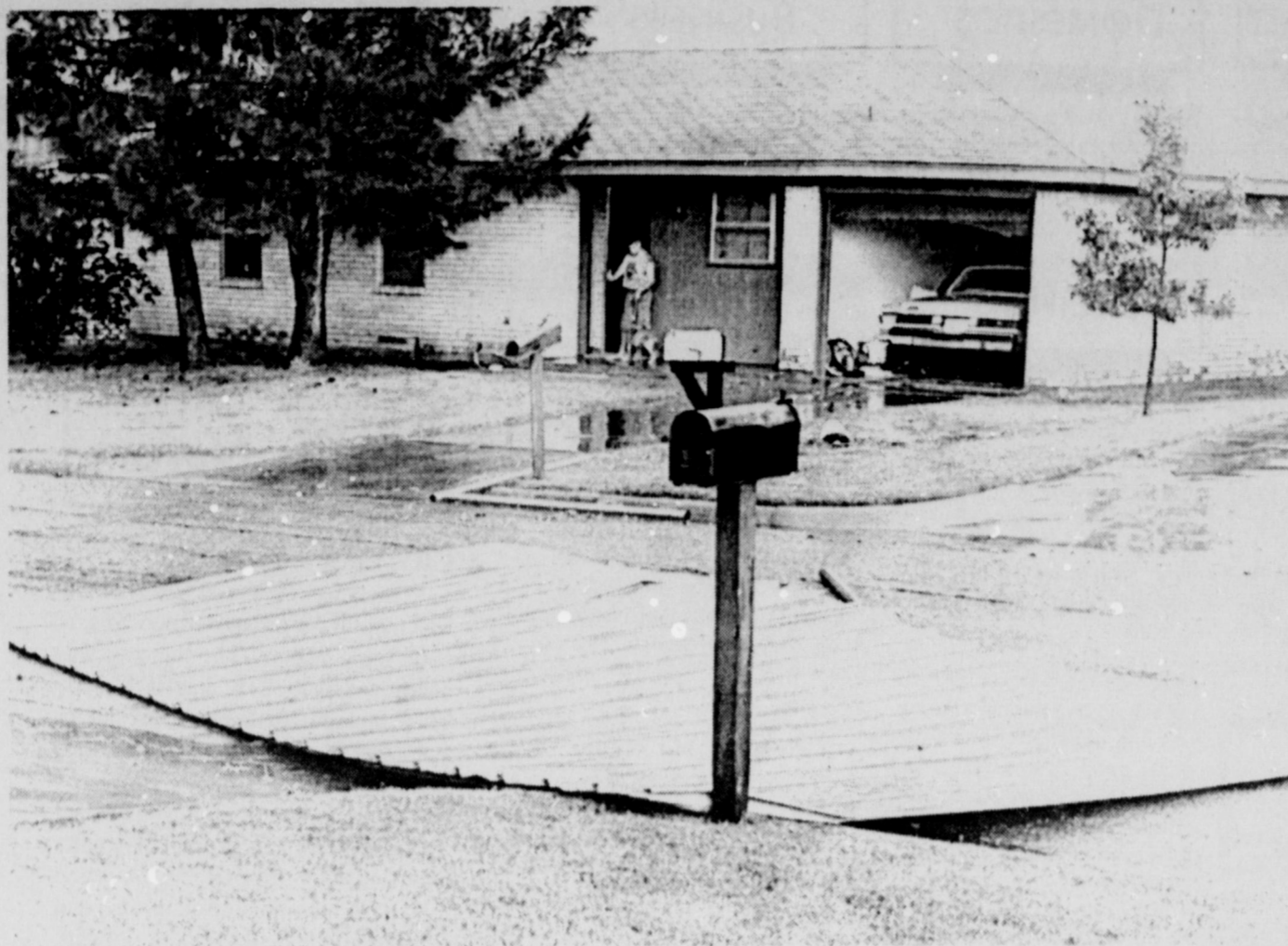
THE REMAINS of a carport covered much of Mockingbird Drive, following the storm Monday afternoon. Observers questioned why the carport would be damaged by a wind out of the south, when the home faced the north, and a carport directly across the street had no damage.
