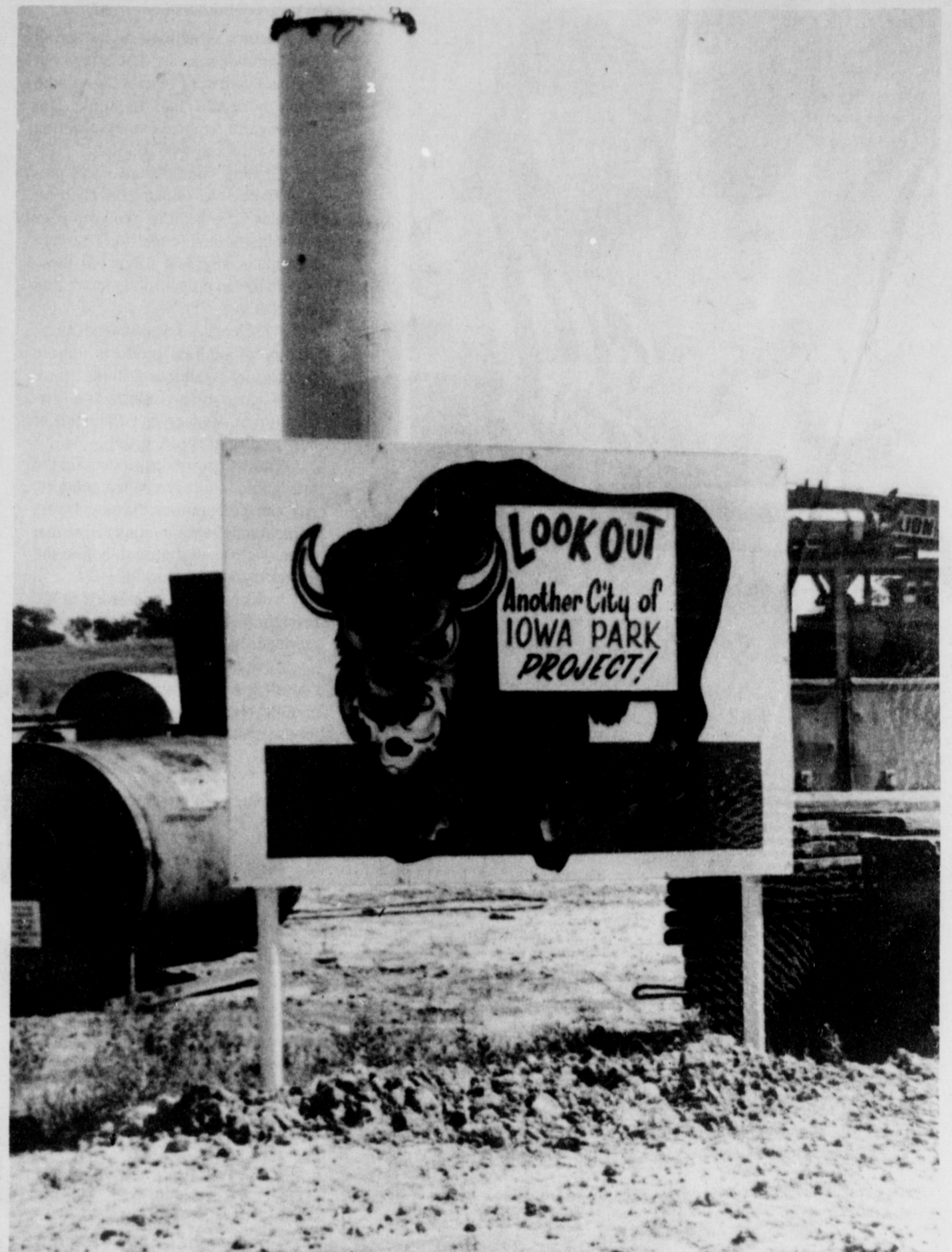
GOING UP! Construction on the new water tower just west of Johnson Road began this week, as crews and materials arrived. The tower's erection is expected to be completed in about three weeks, after which the cleaning and painting process will begin. During that time, water lines are to be laid to connect the tower with areas to the north and west, finally correcting the lower water pressure residents have experienced in recent months.
