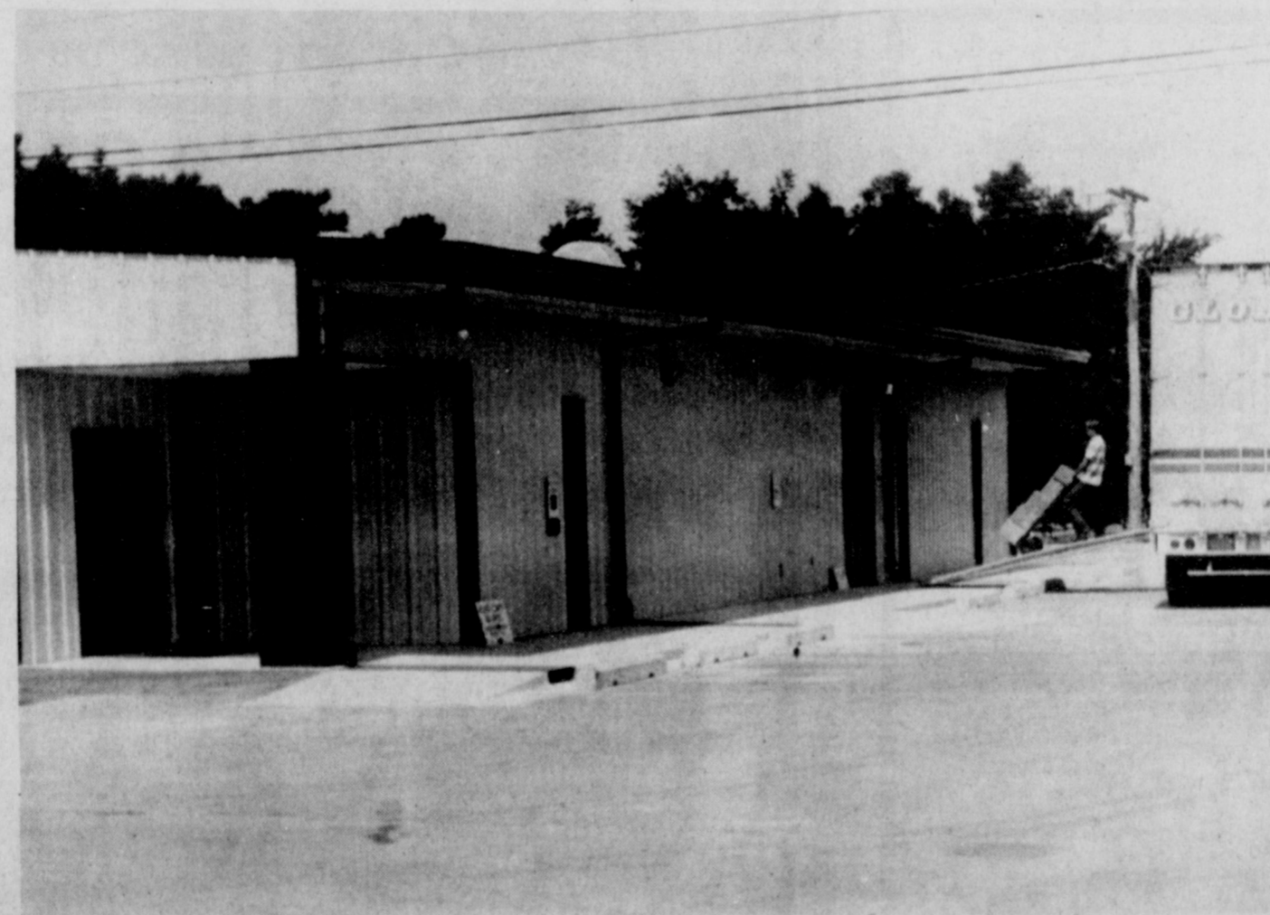
THE BIG MOVE - Occupants of the new county annex building at Bank and Wall began moving Tuesday. They include the Agricultural Stabilization and Conservation, Soil Conservation Service, county clerk's annex and, once a week, the Farmers Home Administration.
