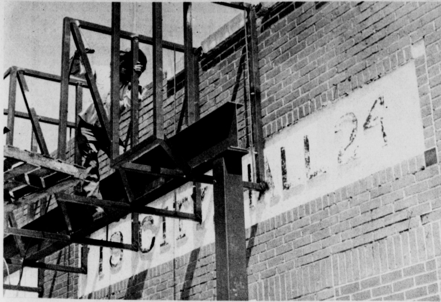
CITY HALL'S COMPLETION in 1924 will no longer be advertised by the sign over the front door, as construction workers this week began erecting substructure for covering the building's exterior. The project is the fourth and final phase of a project initiated some seven years ago.
