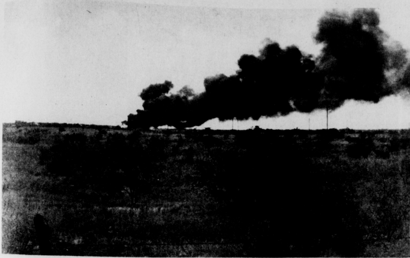
TANK BATTERY FLAMES AFTER BEING HIT BY LIGHTENING
