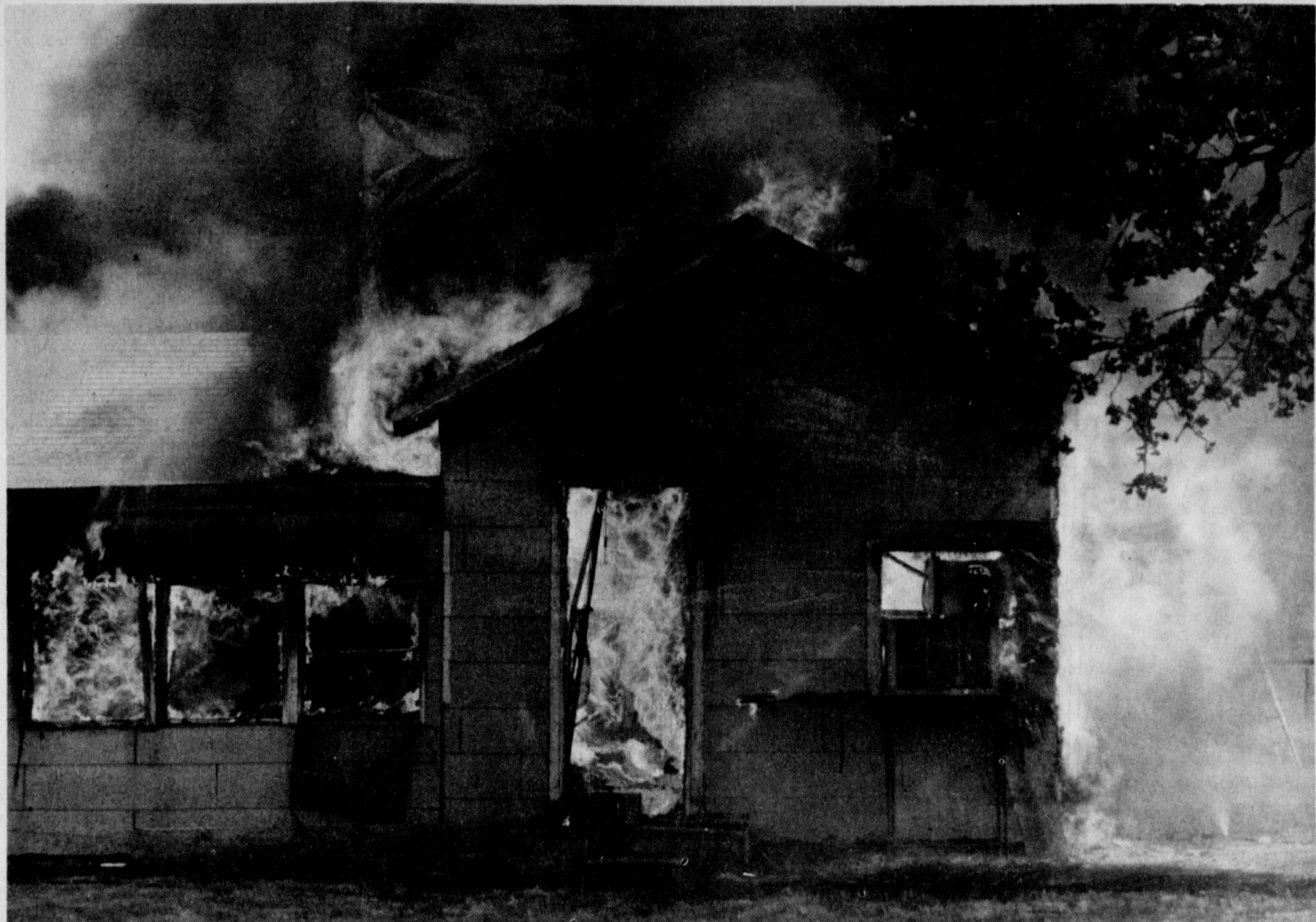
TOTAL LOSS - The home of Carl Fulfer on Coleman Park Road, and all the family's belongings, were lost in a roaring fire Saturday morning. Fulfer said the family was at home when an electrical outlet for the air conditioner, shown on the
