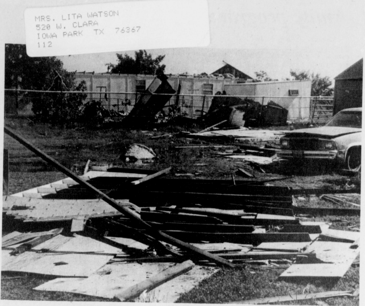
HOUSE ROOF DESTROYED BY THURSDAY NIGHT WINDS ON HUNTINGTON LANE . . . most serious damage reported in the Iowa Park area.
